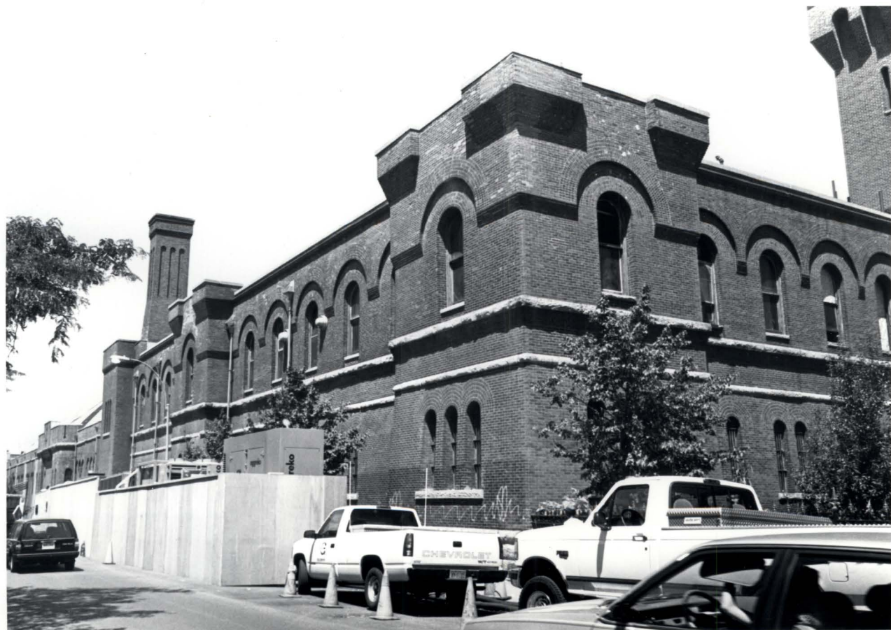
14th Regiment Armory, 1402 Eighth Avenue, Borough of Brooklyn. 15th Street facade, Administration Building. Photo: Carl Forster, 1997.
