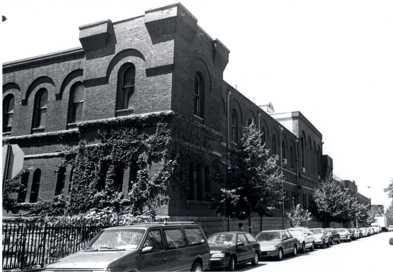
14th Regiment Armory, 1402 Eighth Avenue, Borough of Brooklyn. 14th Street facade, Administration Building. Photo: Carl Forster, 1997.
