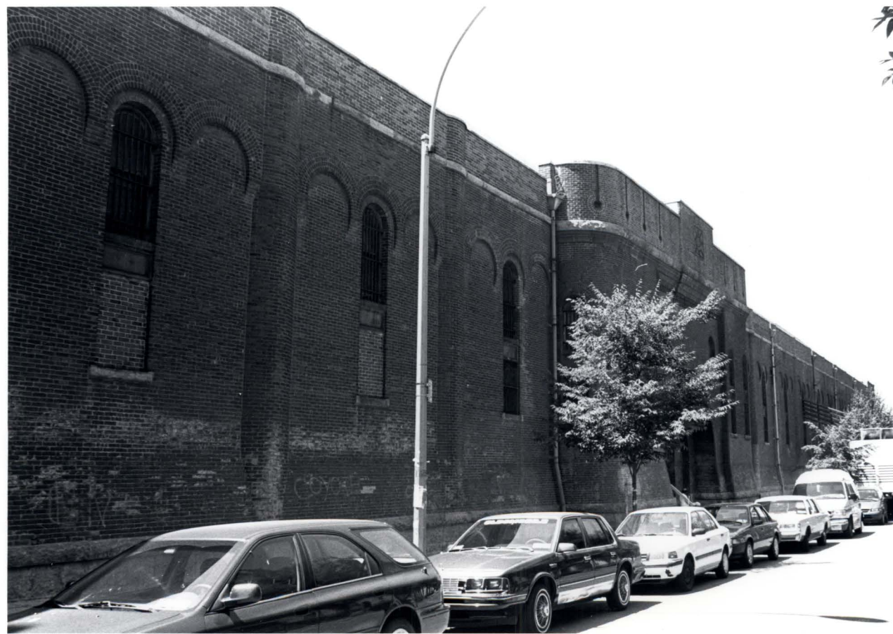
14th Regiment Armory, 1402 Eighth Avenue, Borough of Brooklyn. 14th Street facade of drill shed with sally port. Photo: Carl Forster, 1997.
