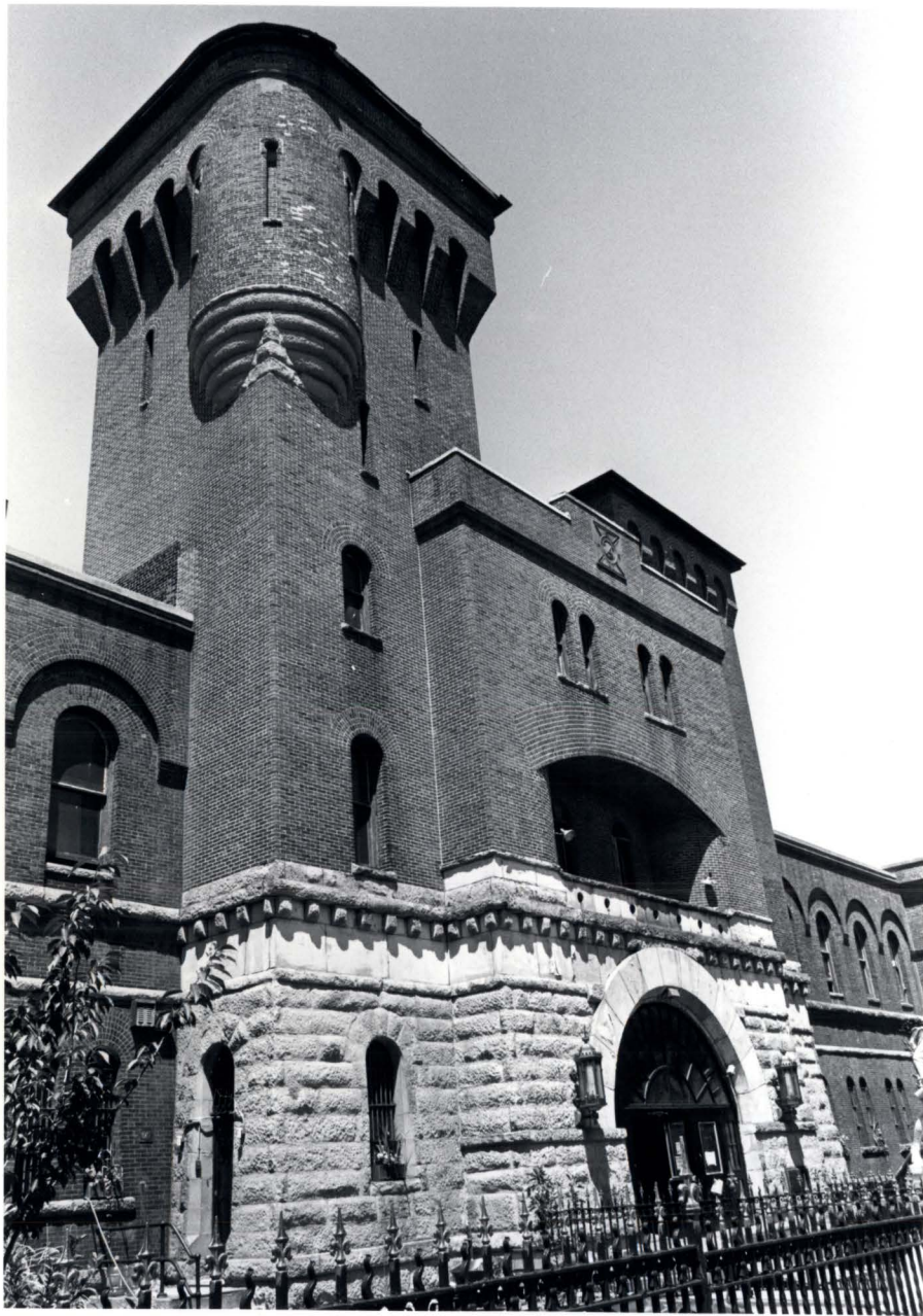
14th Regiment Armory, 1402 Eighth Avenue, Borough of Brooklyn. Eighth Avenue facade with central entrance pavilion and towers. Photo: Carl Forster, 1997
