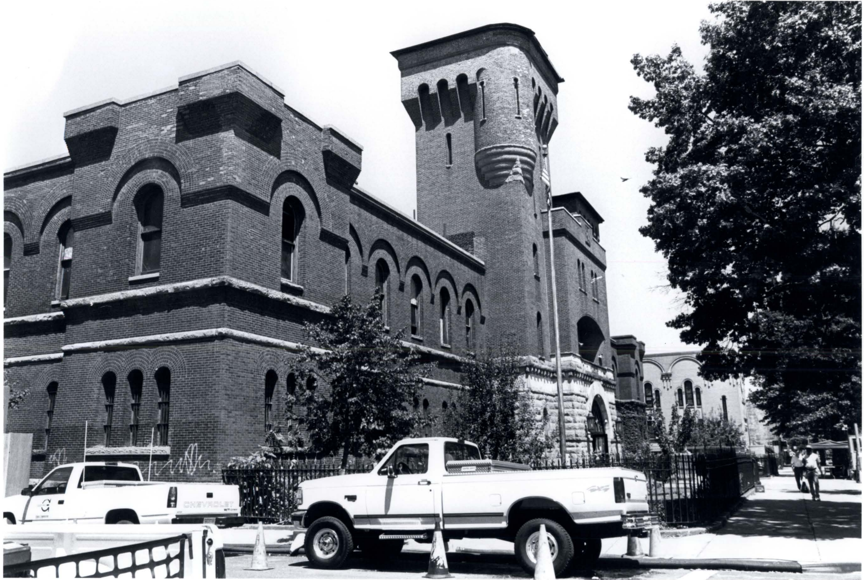
14th Regiment Armory, 1402 Eighth Avenue, Borough of Brooklyn. Administration Building, facing Eighth Avenue Photo: Carl Forster, 1997
