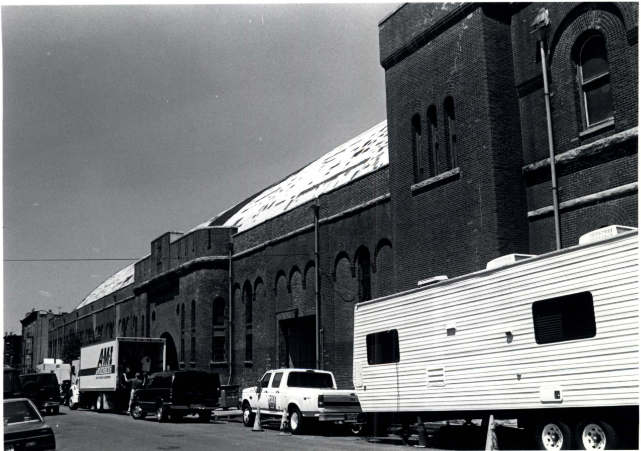
14th Regiment Armory, 1402 Eighth Avenue, Borough of Brooklyn. Eastern end of 15th Street facade, Administration Building. Photo: Carl Forster, 1997.
