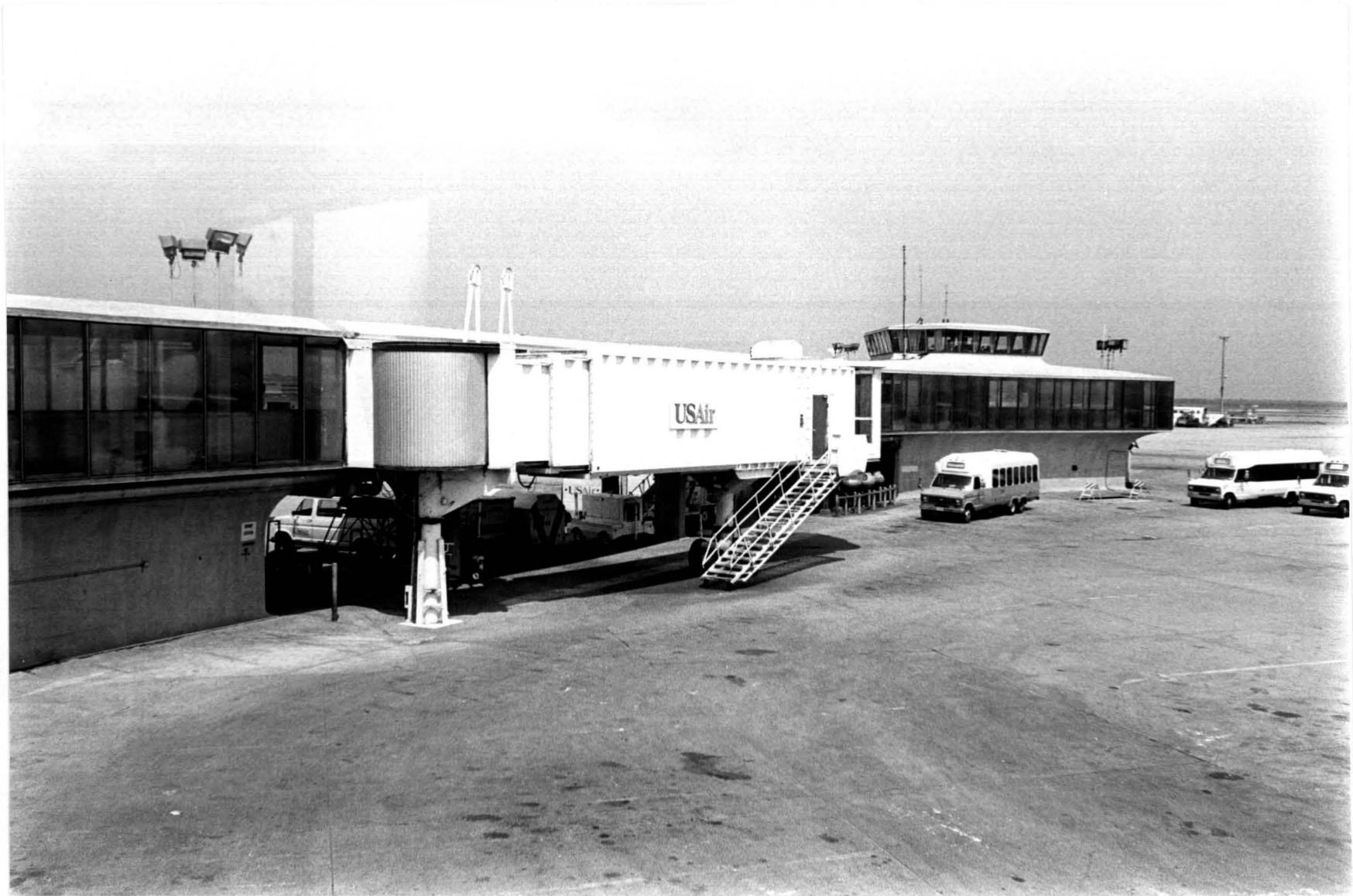
Trans World Airlines Flight Center at New York International Airport. John F. Kennedy International Airport, Queens. East gate structure and Gate 39.
