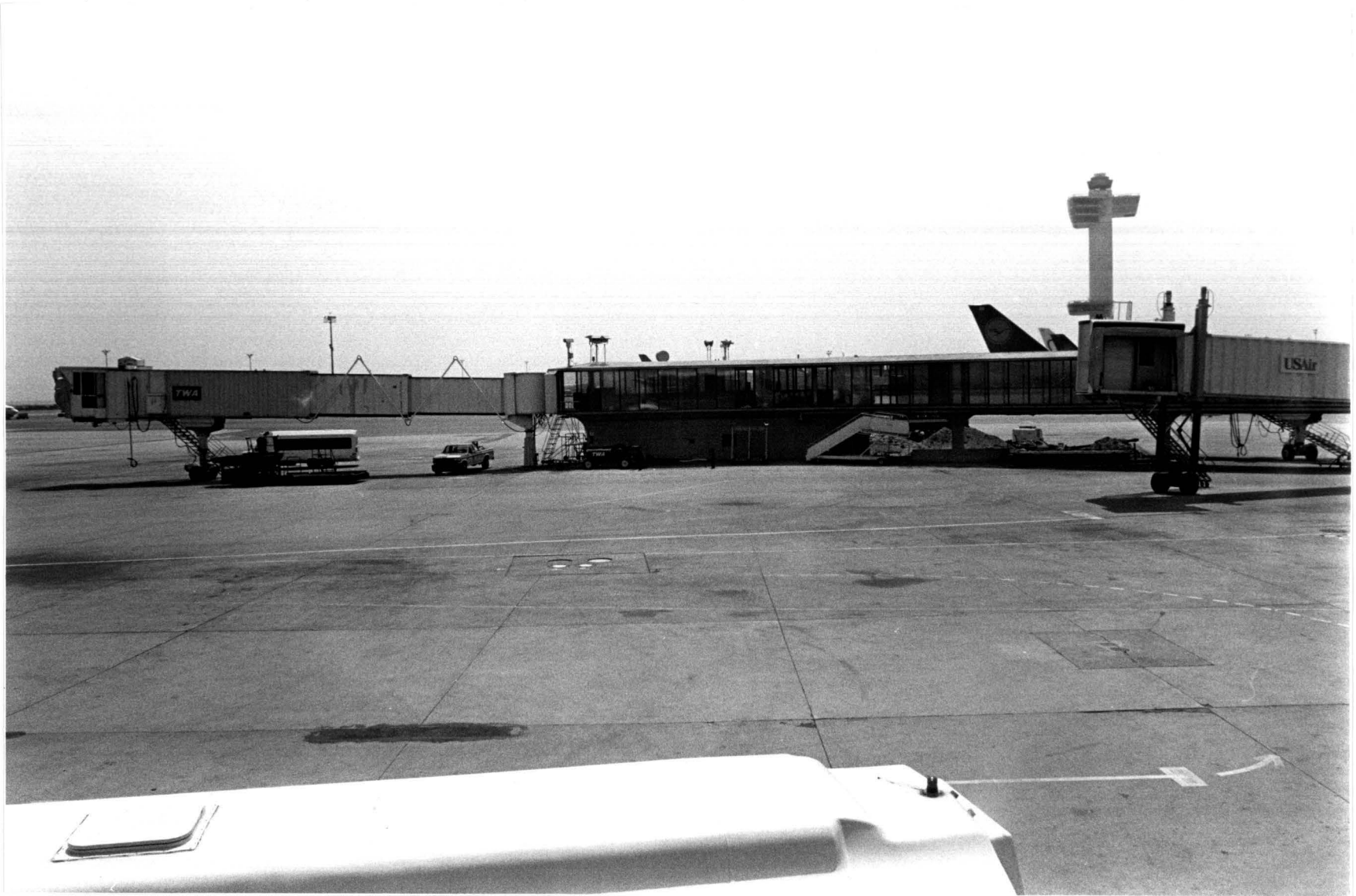
Trans World Airlines Flight Center at New York International Airport. John F. Kennedy International Airport, Queens. Gate 42, east gate structure.
