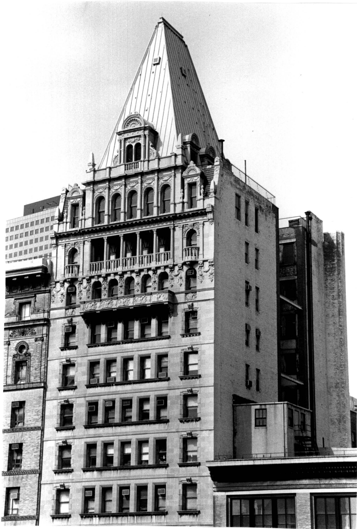
Plate 6. Detail, upper stories and steep roof. Home Life Insurance Company Building. (Carl Forster)
