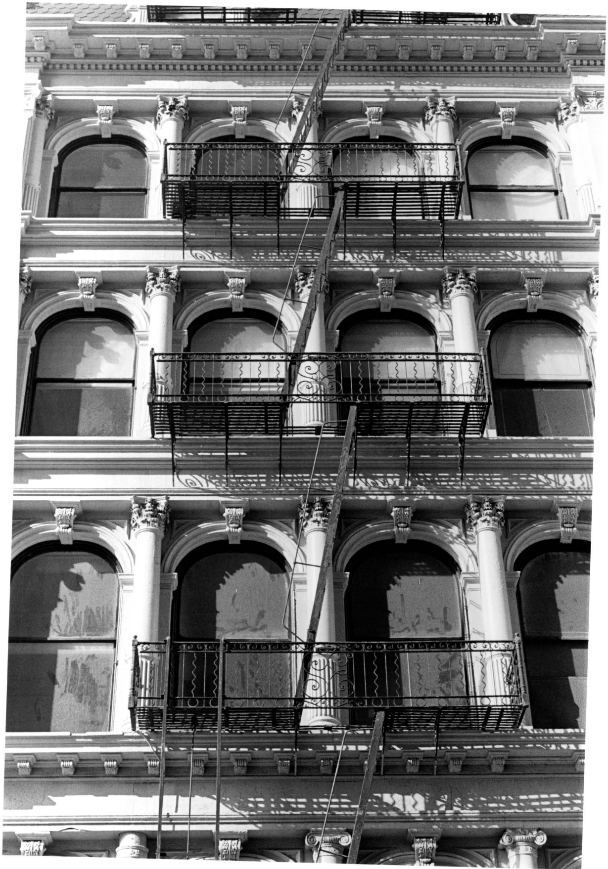
No. 287 Broadway Building
