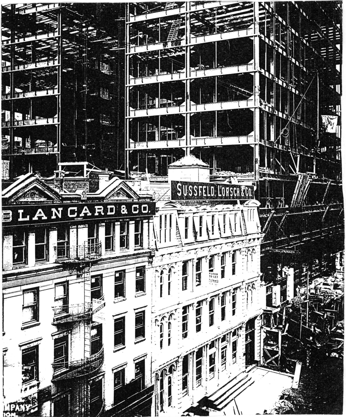
90-94 Maiden Lane Building Historical Photo: October 1911 Showing the mansard roof with its original fishscale slates and segmental pedimented dormers
