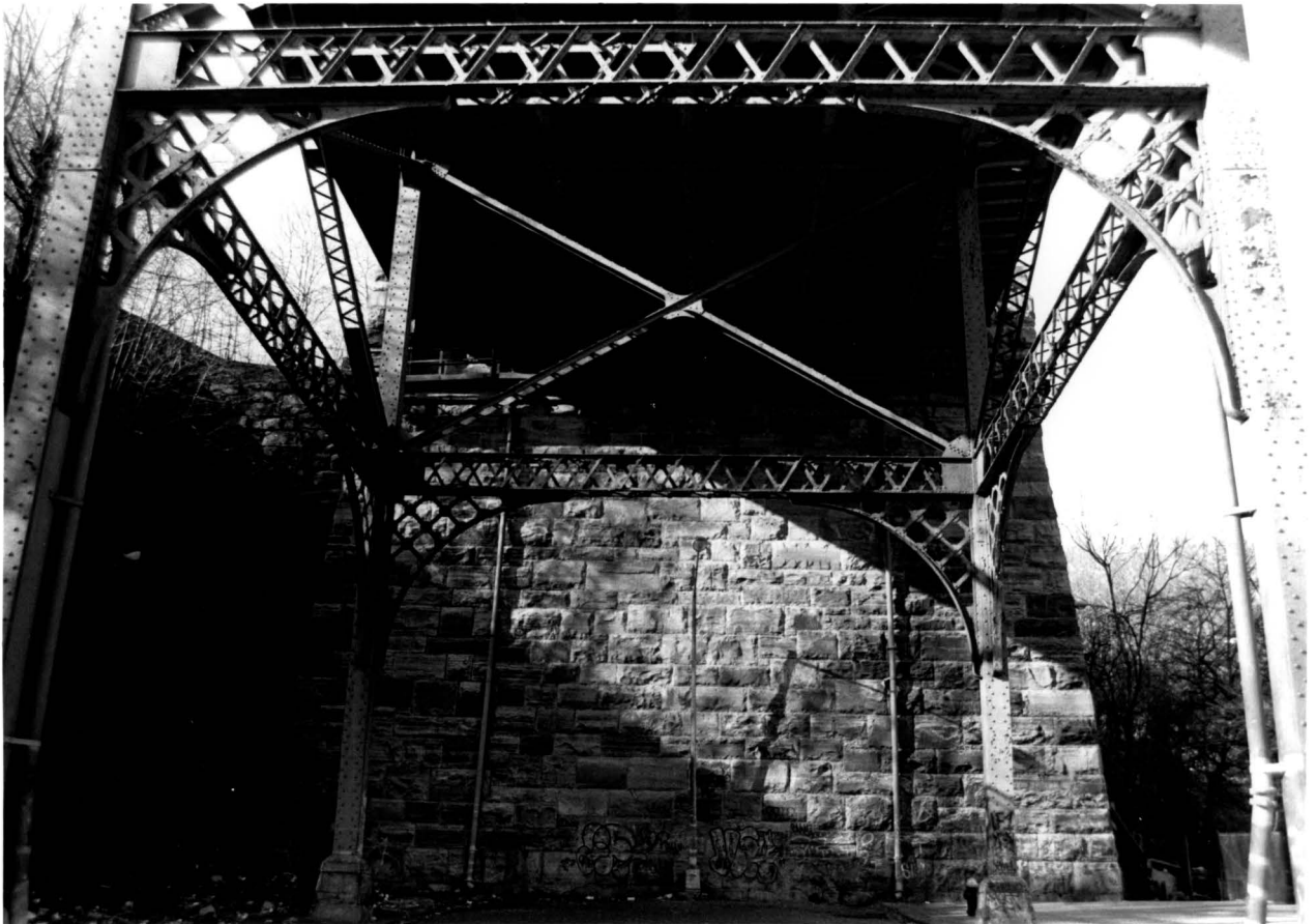
fig. S: 155th Street Viaduct
