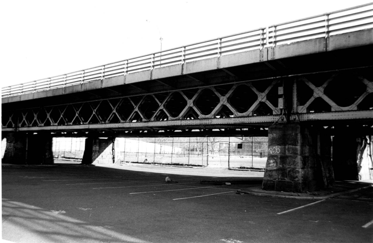
fig. Q: Macomb's Dam Bridge, Jerome Avenue approach camelback truss
