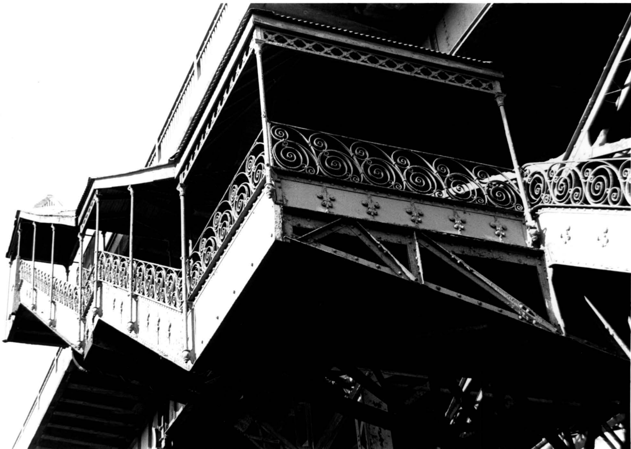
fig. U: 155th Street Viaduct, original railing, west end
