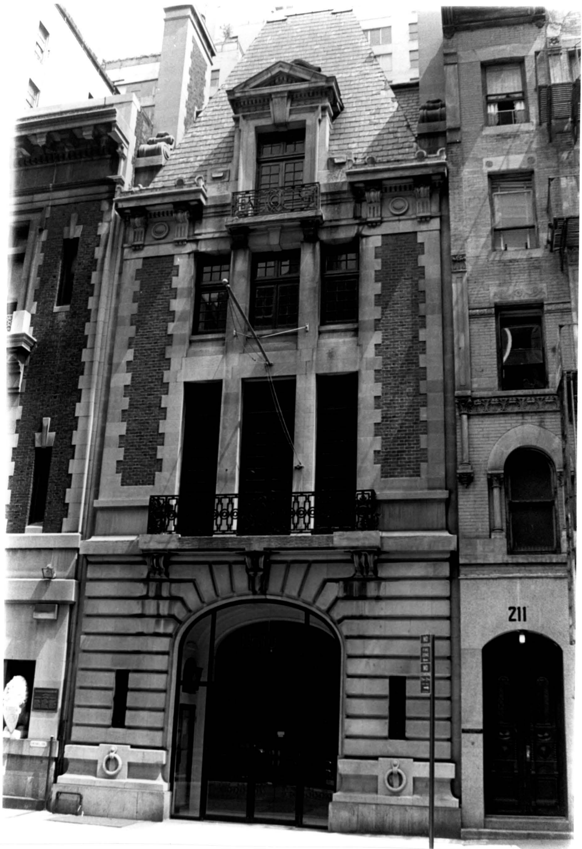
Plate 7. Full elevation, 213 West 58th Street.
