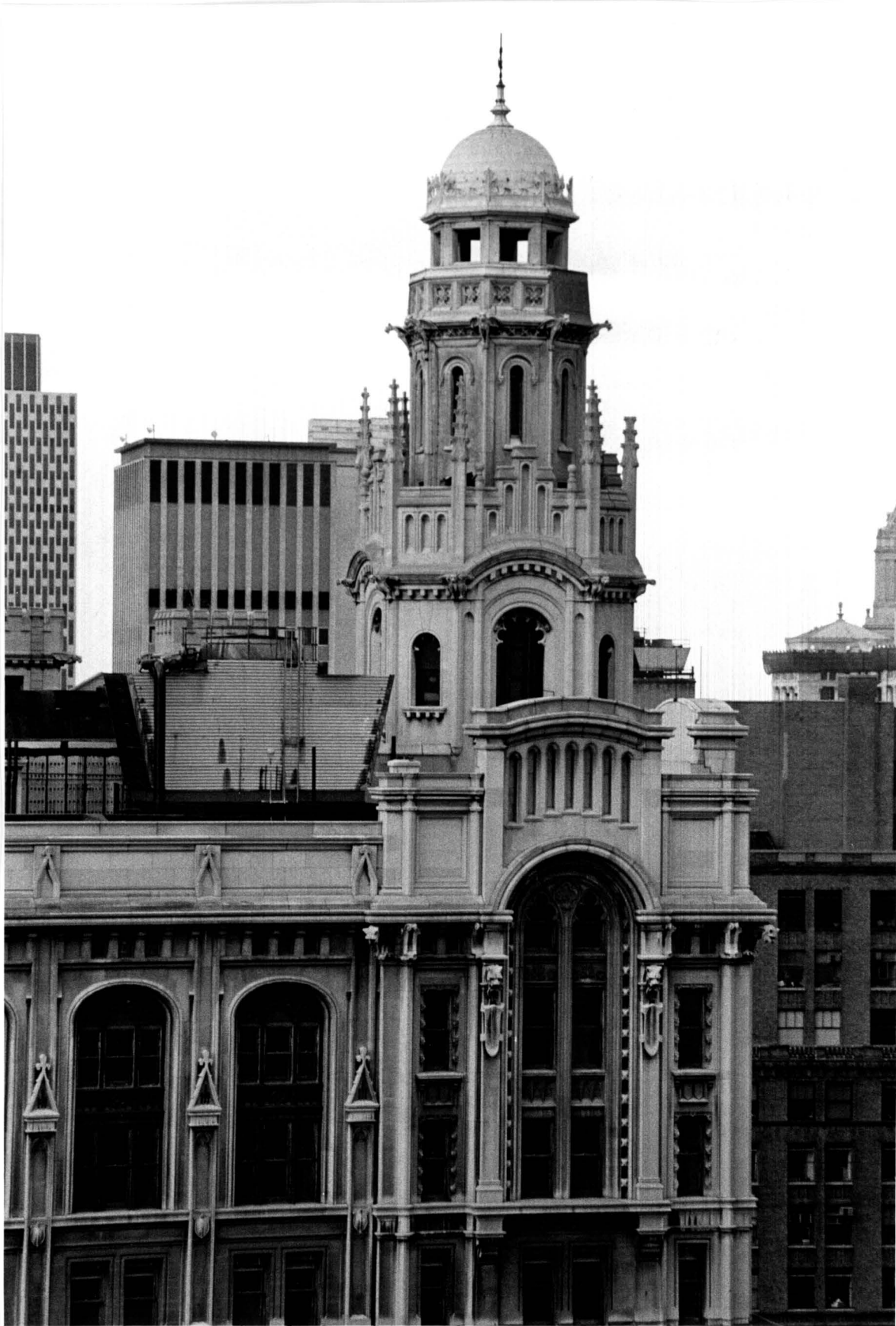
Trinity Building Detail, roofline with cupola
