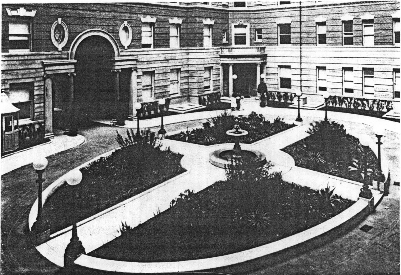
Graham Court Apartments, 1923-1937 Adam Clayton Powell, Jr., Blvd. Clinton & Russell, architects. Built: 1899-1901
