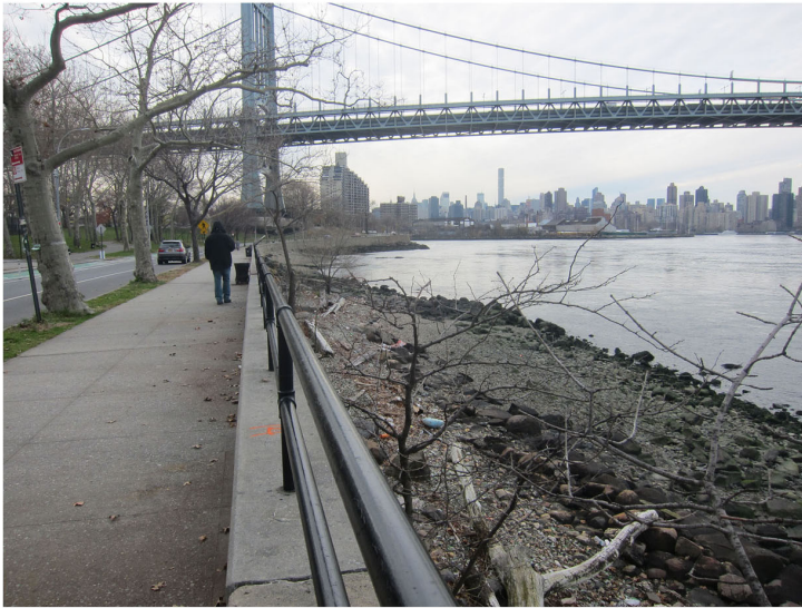
Photo 1. Looking south from the west side of Shore Boulevard. In the far left background, beyond the park, are the tall buildings of Astoria (Pot) Cove development. Protective riprap and the East River beach run below the concrete wall with its pipe fence. (Photo: Geismar 12/8/2016)
