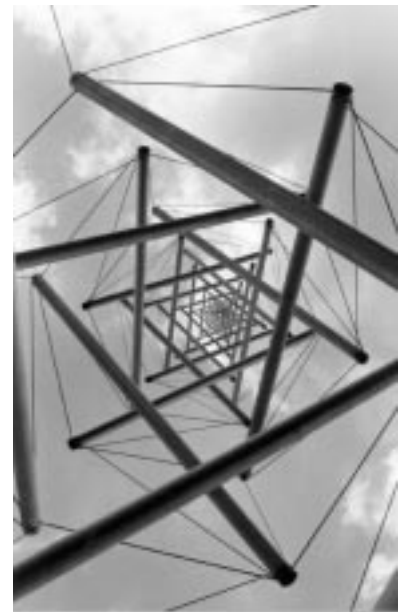
Figure 4.27: Sometimes trusses are used only because they look nice. The tensegrity structure 'Needle Tower' was designed by artist Kenneth Snelson and is on display in the Hirshhorn Museum in Washington, DC. Here you are looking straight up the middle. Photograph by Christopher Rywalt.
