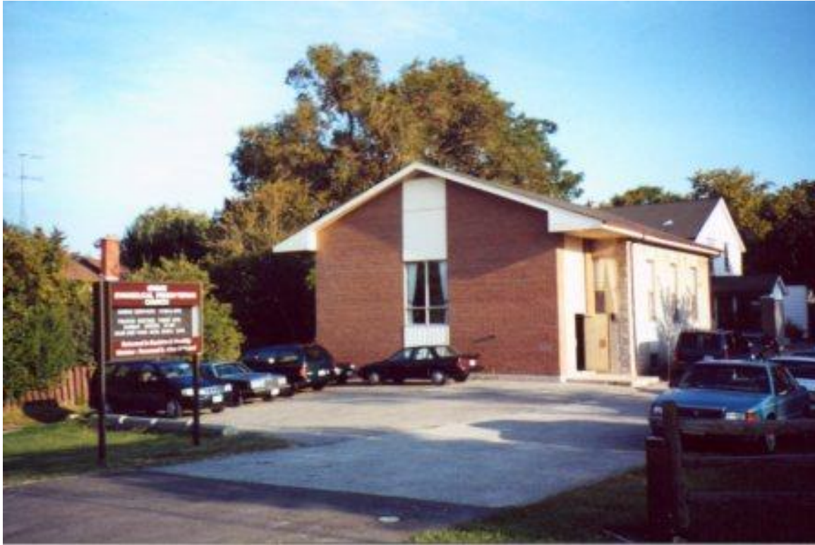
593 Sheppard Ave. East before the Subway Construction Commenced
