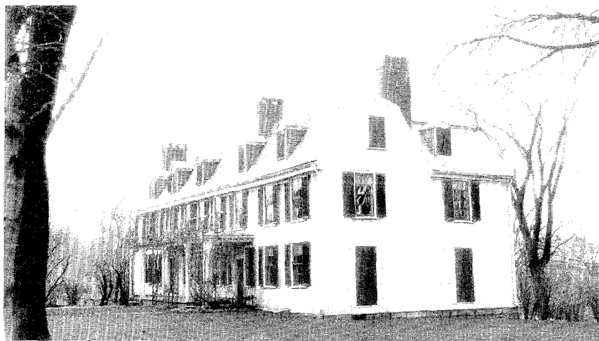
PHOTOGRAPH OF OLD HOUSE WITHOUT EASTERN PORTICO, A.F. SHURROCKS PHOTOGRAPHY CO., 1928.
