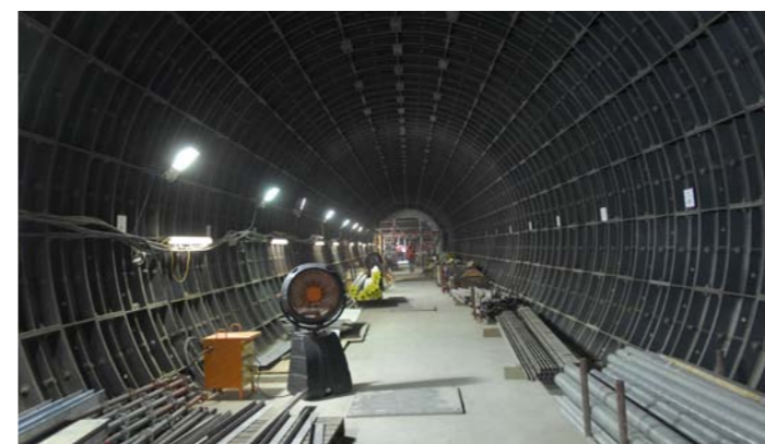
Tunnels: 300m of new tunnels were excavated and fitted out
