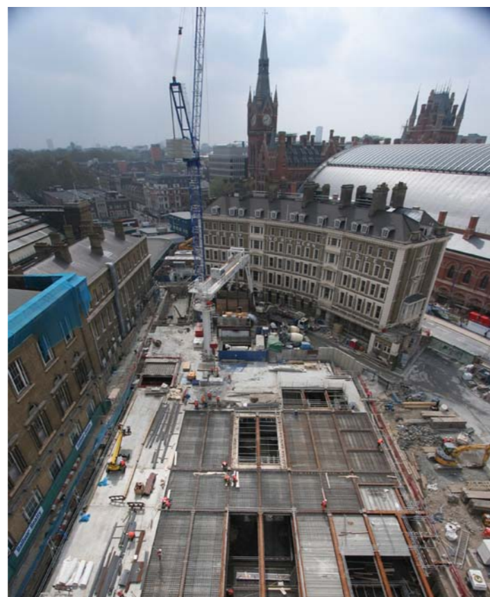
Slab: Materials were delivered through openings in the concrete roof
