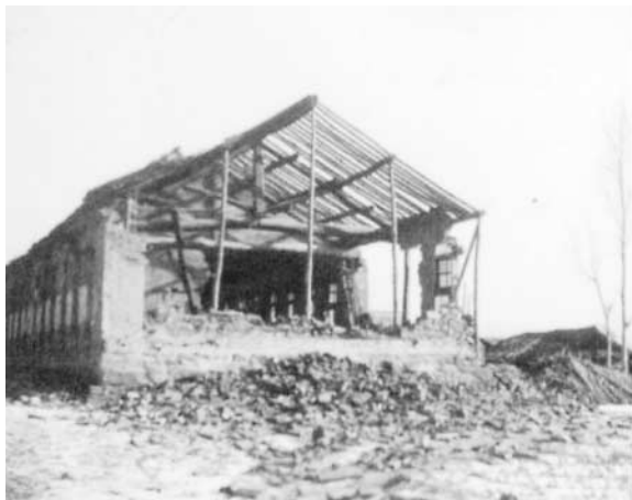
Figure 9. Examples of damaged or collapsed houses in Haicheng County to show the shake-resistant nature of their wooden frames. Left: Chagou Commune. Right: Ganwang Commune. See Figure 6 for locations of the communes.
