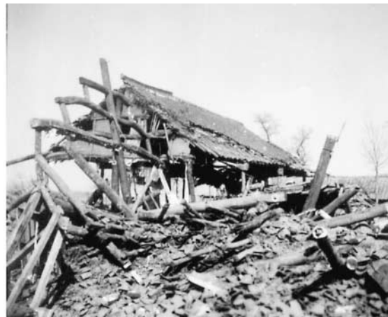
Figure 9. Examples of damaged or collapsed houses in Haicheng County to show the shake-resistant nature of their wooden frames. Left: Chagou Commune. Right: Ganwang Commune. See Figure 6 for locations of the communes.
