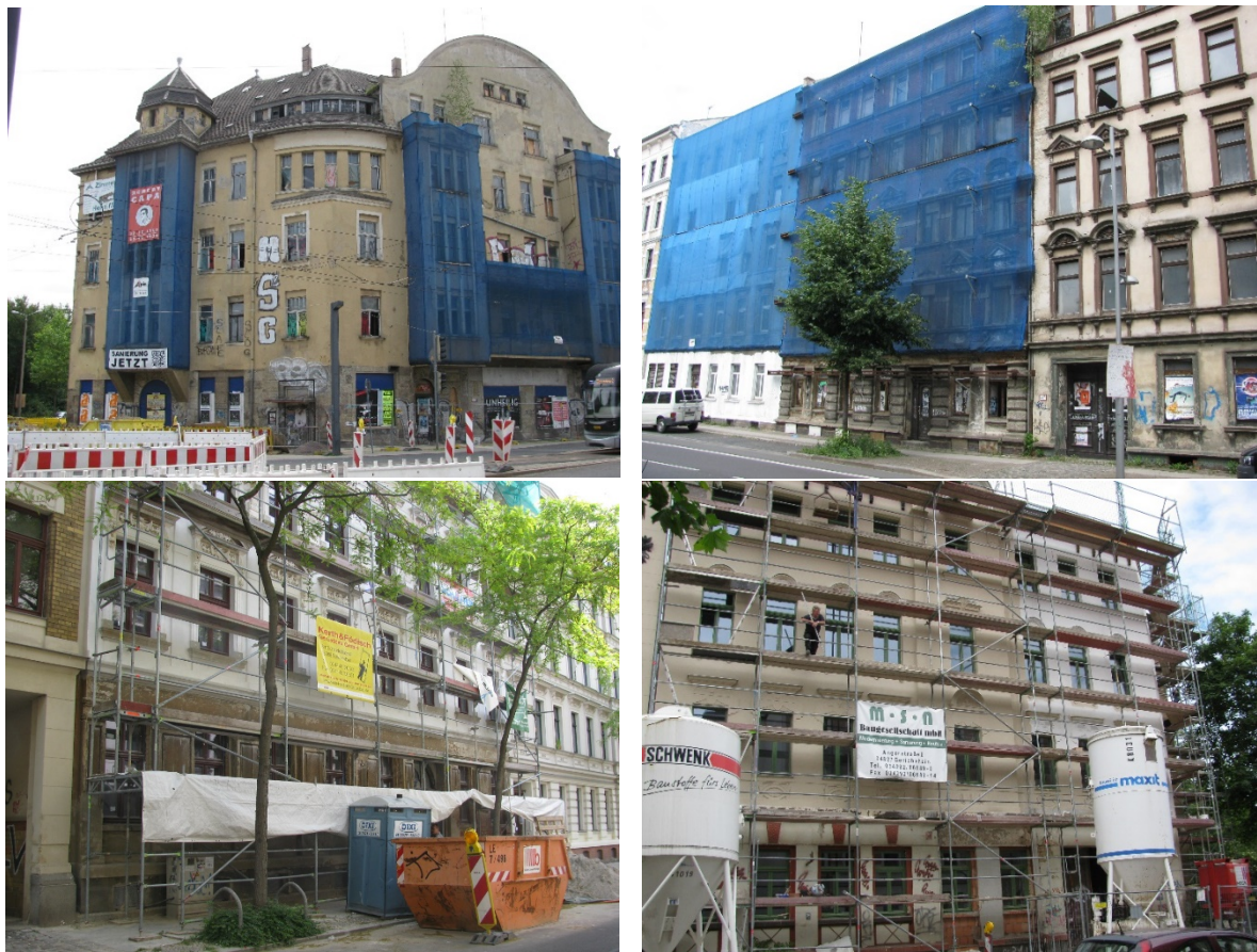
Figure 37: Buildings being renovated and for sale
