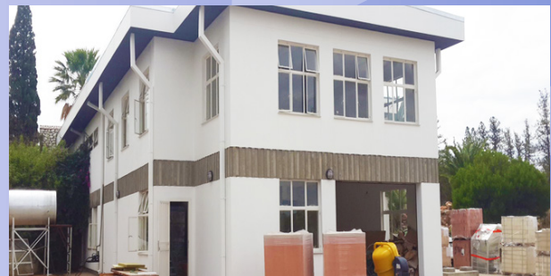
Upgraded Windhoek Crematorium
