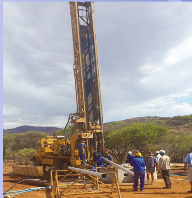
Deep drilling of water boreholes
