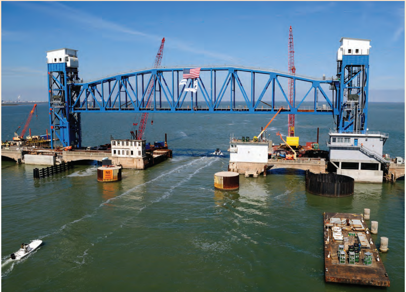
Figure 4 – Galveston Island Railroad Bridge.
