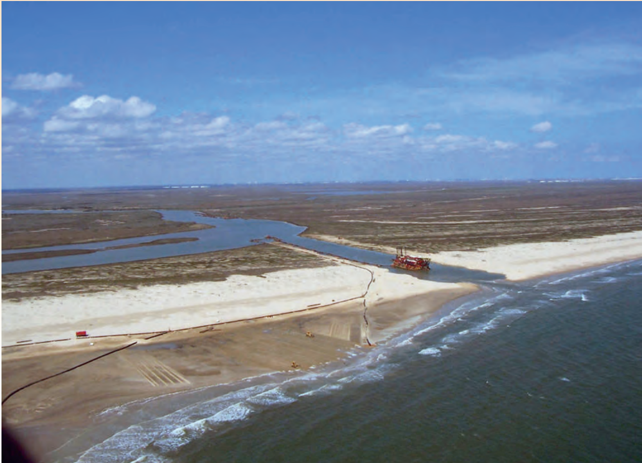
Figure 3 - San Bernard Dredging Project.
