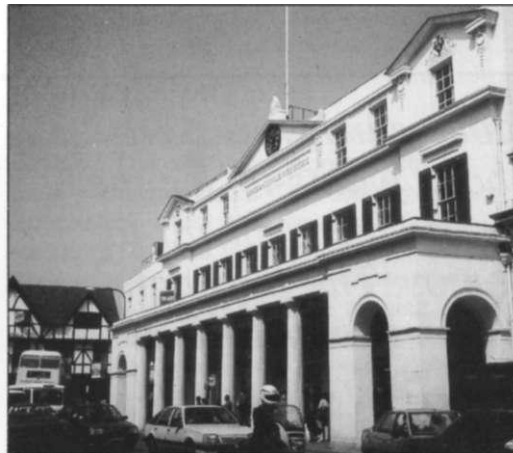
This grand frontage, built in 1820, belonged to a company which also looked after people and their property — the Essex and Suffolk Insurance Company. The columns are made of cast iron.
