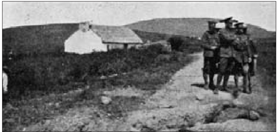
A trenched road near Ballymote (Dunnill, Summary)
