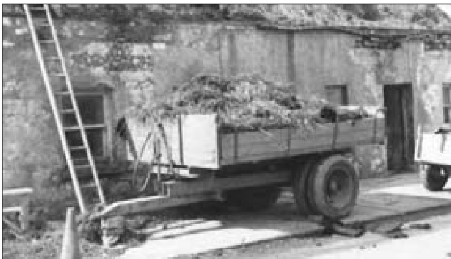
Thatched cottages in Mill Street photographed by Maisie McGovern before demolition in 1979/80 for construction of new house by Tom Currid for the Coleman family.
