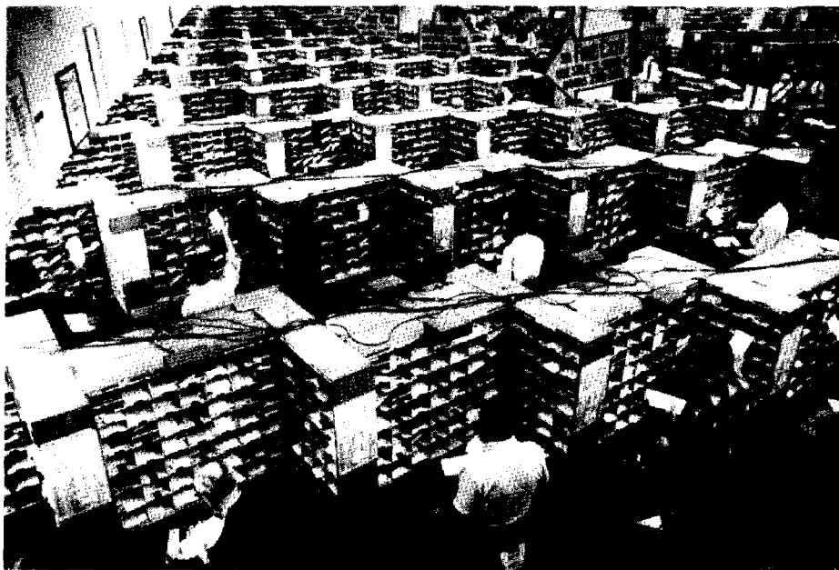
Using manual "pigeon hole" method, clerks can sort up to 800 pieces of mail per work-hour. (U.S. Postal Service photo)
