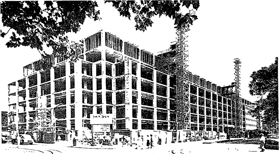
Construction Progresses Further. GAO Building, September 1950.
