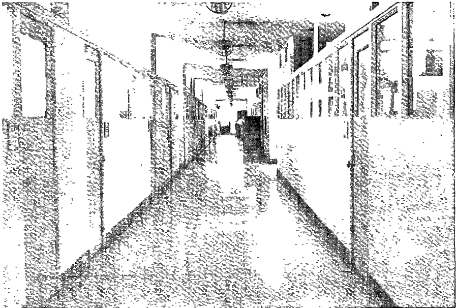
Typical corridor before renovation.
