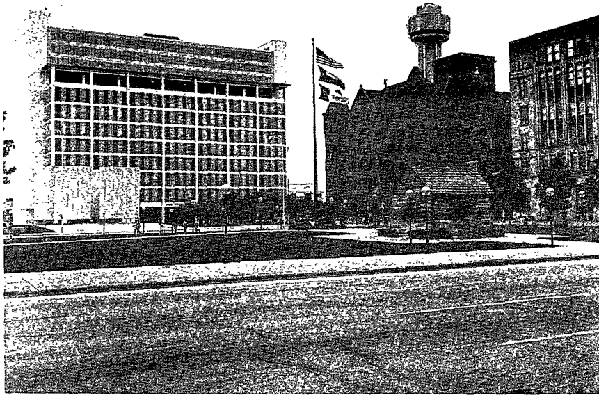
County Court House Plaza, the old and new, downtown. John Neely Bryan cabin, Dallas' first building and first courthouse (1841) stands in view of the newest addition to its already impressive skyline, Reunion Tower (1978). Behind the John F. Kennedy Memorial (left foreground) is the present county courthouse (1968) and behind the cabin the "old" county courthouse (circa 1890).
