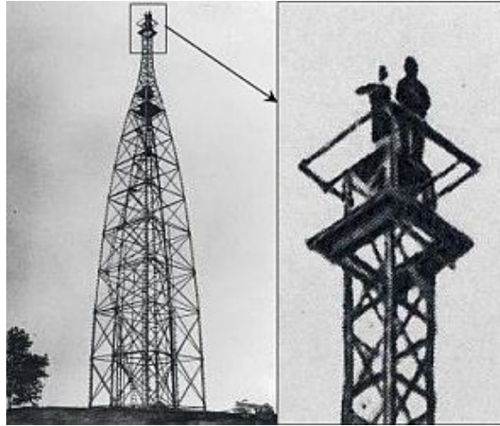
Figure 3.1: Observing towers called Bibly towers built for triangulating other towers. Figure courtesy of (Natural Resources Canada, 2009).
